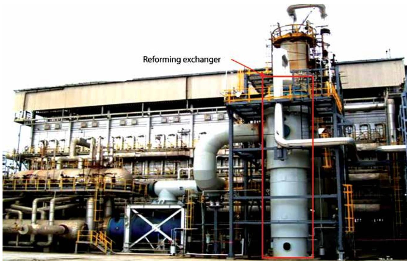
Figure 1. KRES in operation in CFCL ammonia plant.
